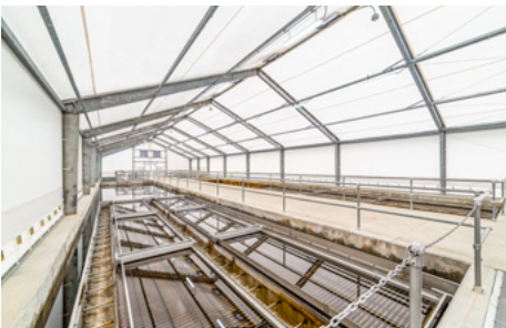
Water & Wastewater Treatment Facilities
