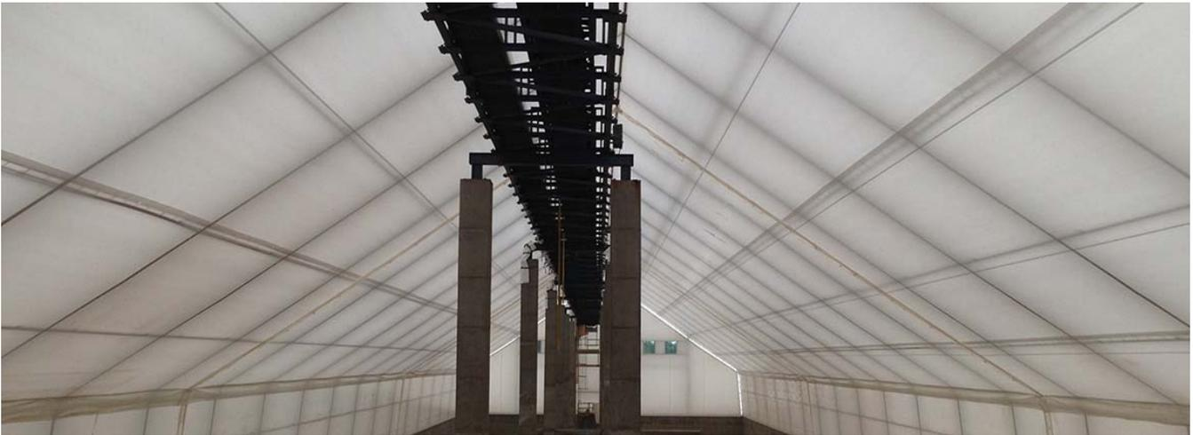
Figure II: Interior liner to protect the steel frame
