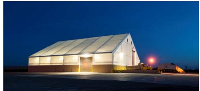
Figure V: Salt storage fabric structure
