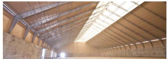
Figure III: Hot dip galvanized steel members
